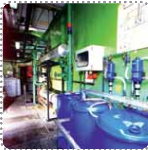
Dosatron installation
